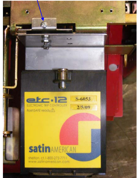
FIGURE 1, PROGRAMMER MOUNTING BRACKET INSTALLED ON BREAKER
