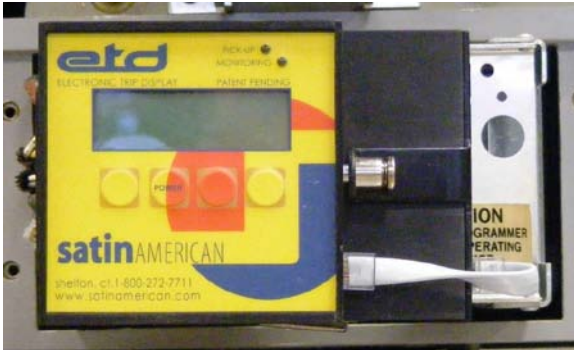
FIGURE 19, etc-12 INSTALLED ON BRACKET
