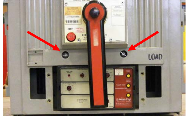
FIGURE 11, REMOVE INDICATED SCREWS
