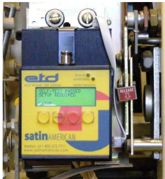
FIGURE 7, NEW UNIT INSTALLED ON BREAKER
