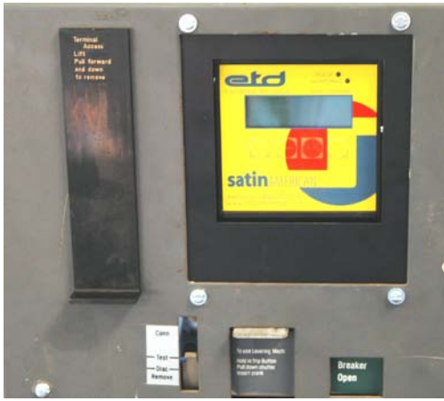
FIGURE 5, etd Installed with windowed escutcheon plate
